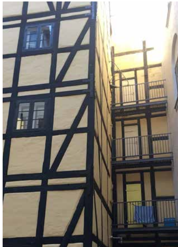
Courtyard building of half timber construction. Photo by the author.
